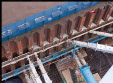
Trench Sheets & Sheet Piles
