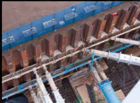
Trench Sheets & Sheet Piles
